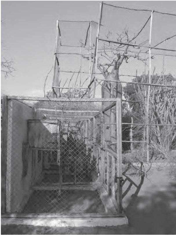
Fig 4: Original LRC enclosures that were built in 2011. Small cages are in the foreground and the large enclosure is in the background.
